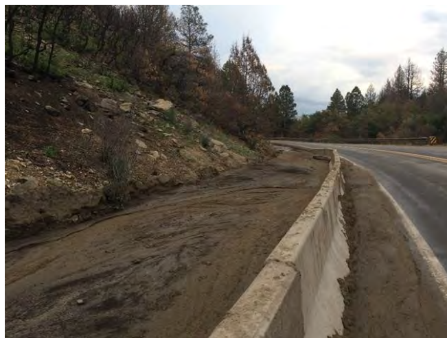
The New Mexico Department of Transportation utilized concrete K-rails to reduce sediment washing off the Ute Park Burn on Highway 64 west of Cimarron, NM. © Mary Stuever/NMFD
