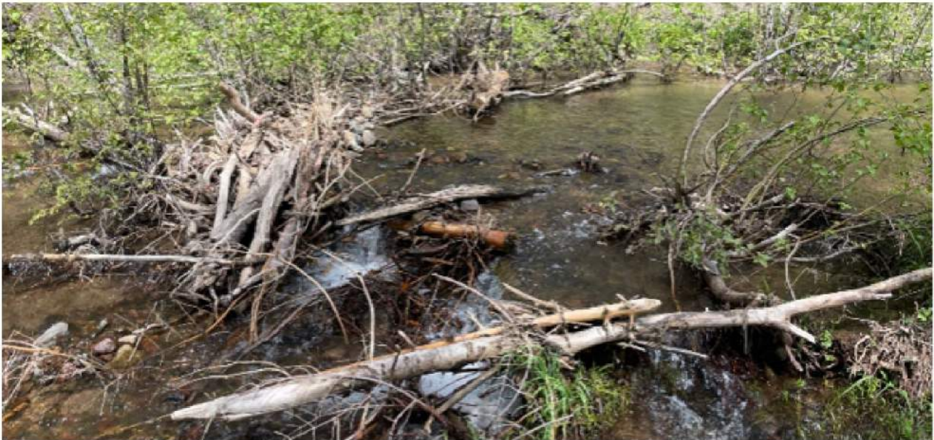
Riparian beaver dam analog structures in Rio Arriba County. By slowing the water down with structures that emulate beaver dams, habitat is created and the water table is raised up.
